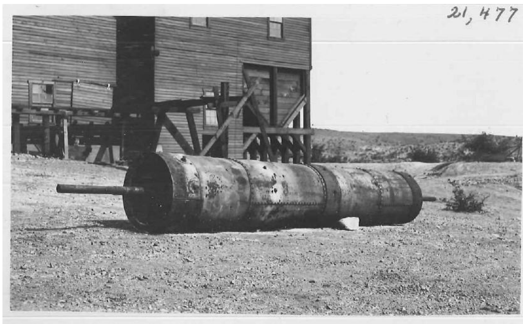
Figura VI.2: Secadora empleada en The Cananea Consolidated Copper Company
